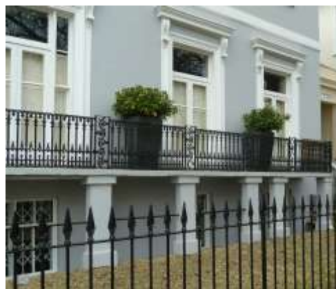
Frontages were adapted to allow more light into basements.
