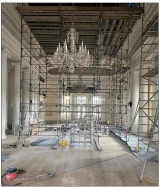
the basement ceiling to ensure that the Pump Room floor could support the weight of the scaffolding required to carry out the repair works. Specialist plasterers are carrying out the repairs which are programmed to take between four and seven weeks, with the re-opening of the Pump Room scheduled to take place in the week commencing 11 March, ahead of the Cheltenham Festival Race Week.'
